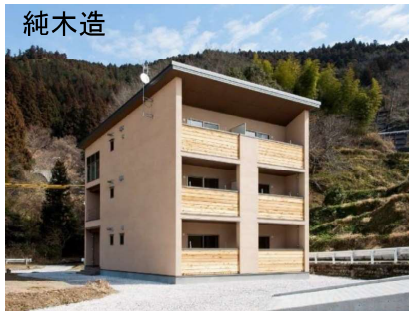
Company dormitory 2014 3story
